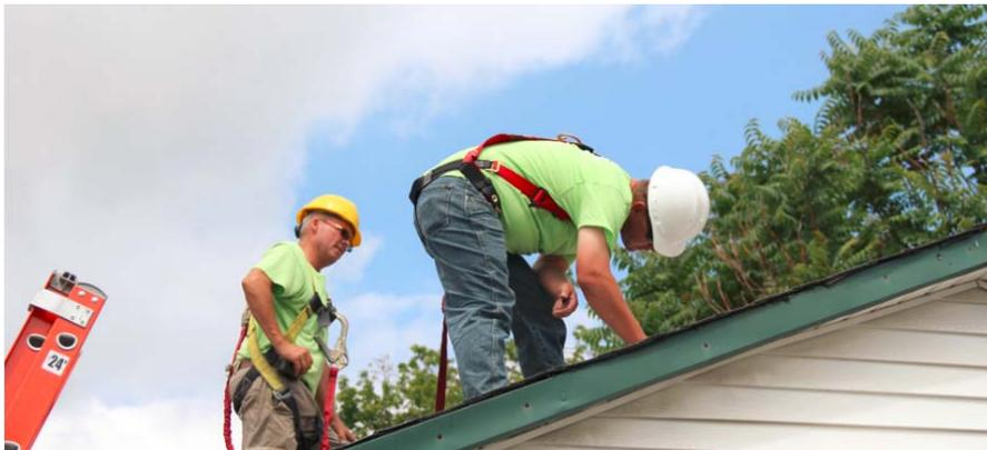
**Figure 3-3: Wearing safety harnesses by all roof workers is one of several safety protocols followed by the contractor's field installation crews.**
